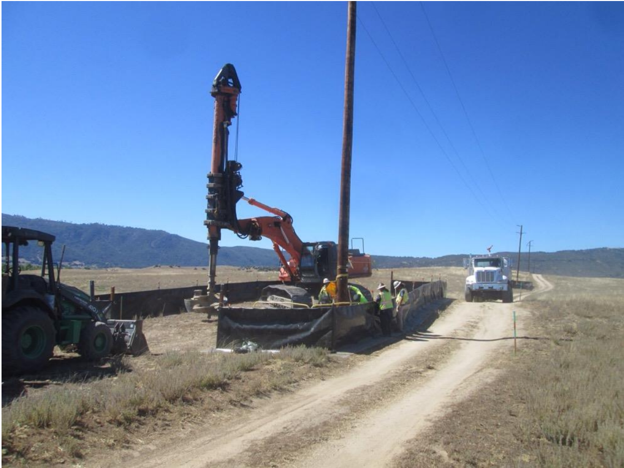
Photo 4: Cultural resource monitors were onsite to inspect excavated spoils during pole hole drilling at Z118208 (TL 682) in accordance with MM CUL-1.
